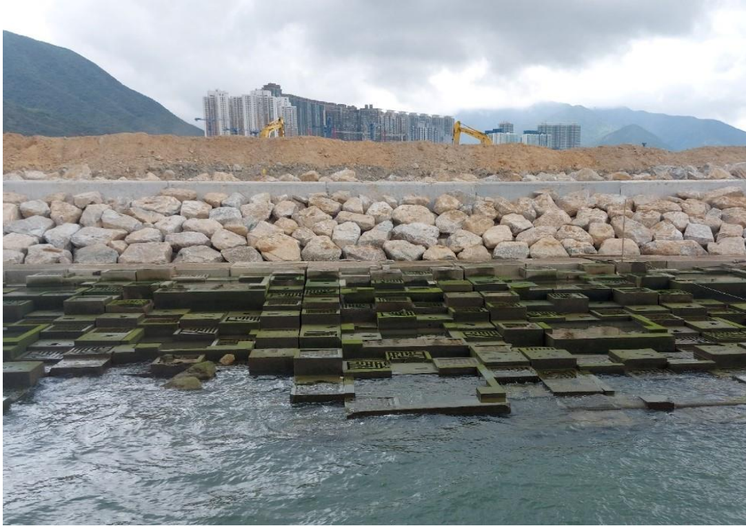
Photo 4 – Natural Rock Material/Planting for Artificial Seawall
