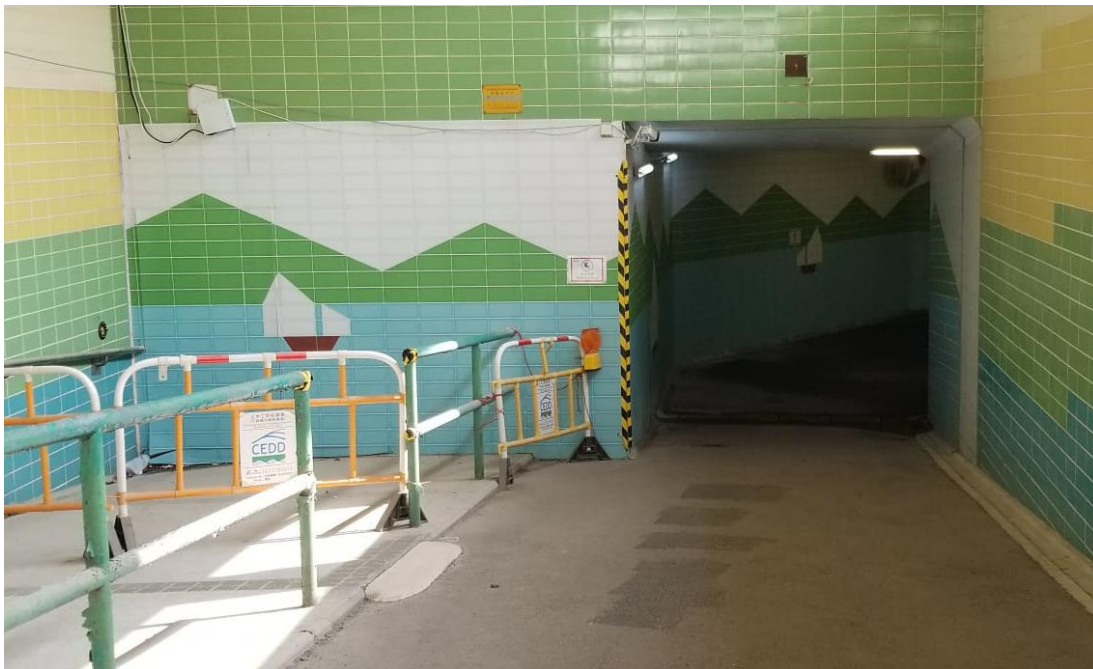
Photo 3 - Erection of site hoardings in unobtrusive colours
